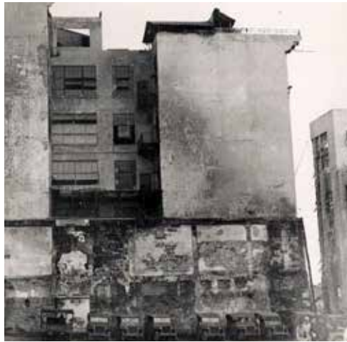
The China Bank Building was partially burned during the war. When the Bank reopened after Manila's liberation, the building was rehabilitated and two more levels were added.
