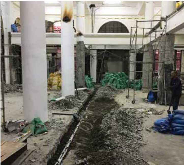
Perforated pipes were installed to collect water and prevent seepage during high tides.
