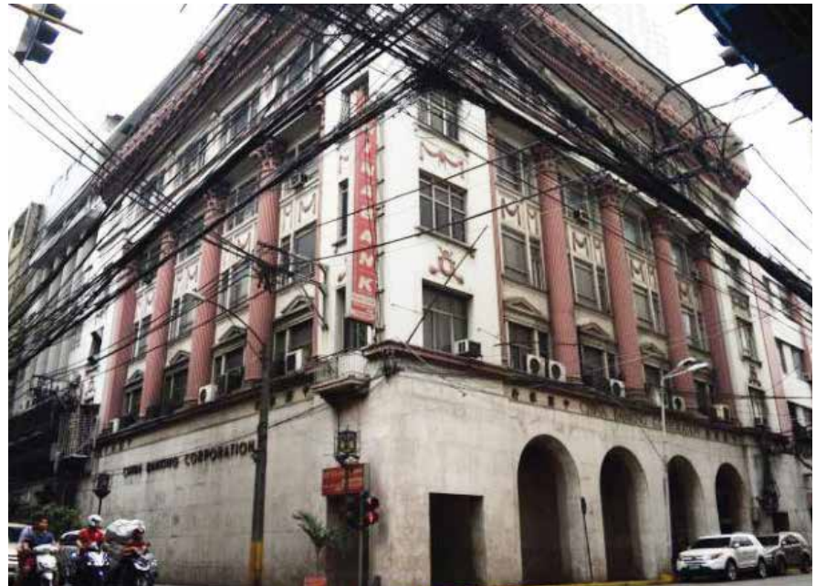
Prior to the restoration, marble cladding installed in the 1960s covered the arches along Juan Luna Street and the internal arches along Dasmarinas Street.
