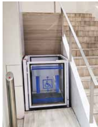
Better access to the safety deposit box (SDB) on the mezzanine floor with a PWD lift.
