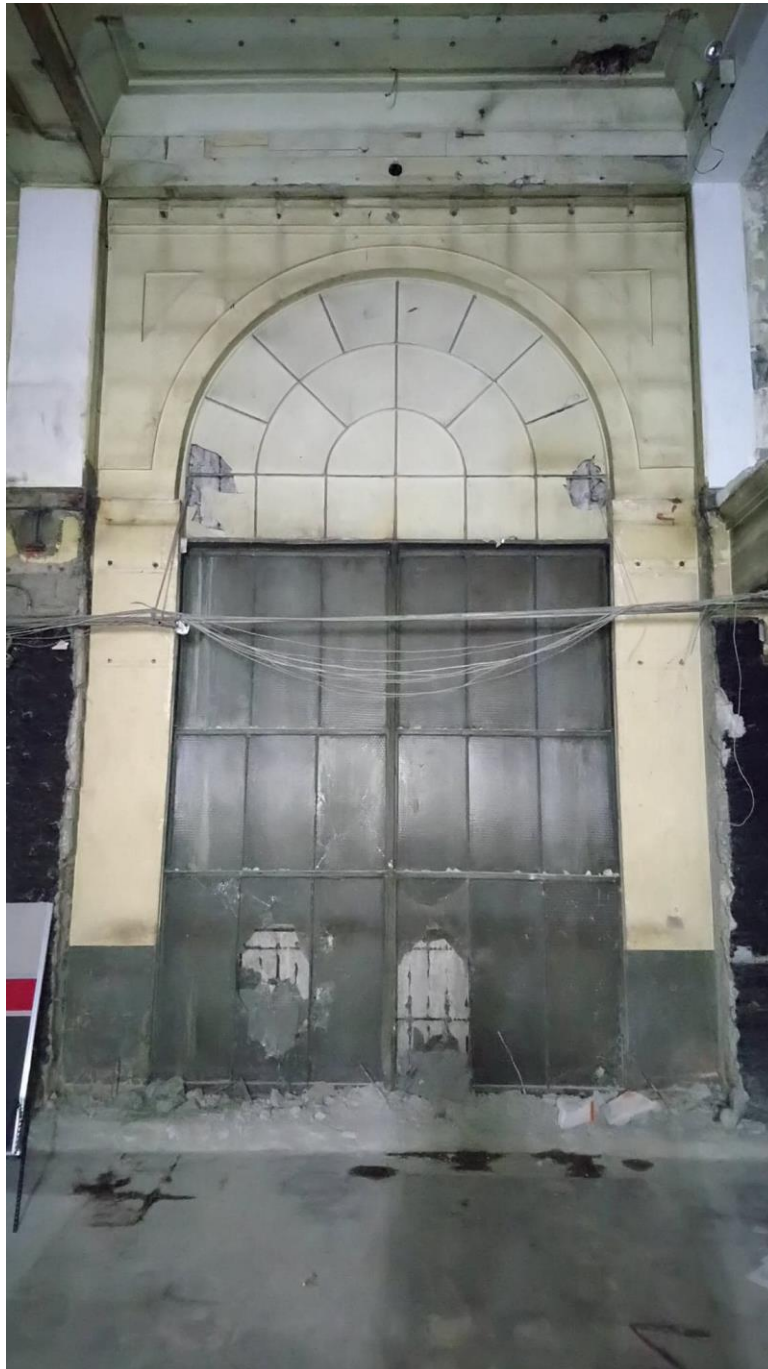
The second arch from the corner of Calle Dasmariñas and Juan Luna along Calle Dasmariñas. The opening is framed by a metal casement with Double Hung Windows. The upper arch is protected by \frac{1}{4} thick glass on a metal frame. Protecting the opening are grillwork's, covered with thick cement.
