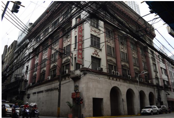
The façade of China Banking Corporation Binondo Business Center prior to renovation with the cladded marble hiding all historic architectural elements
