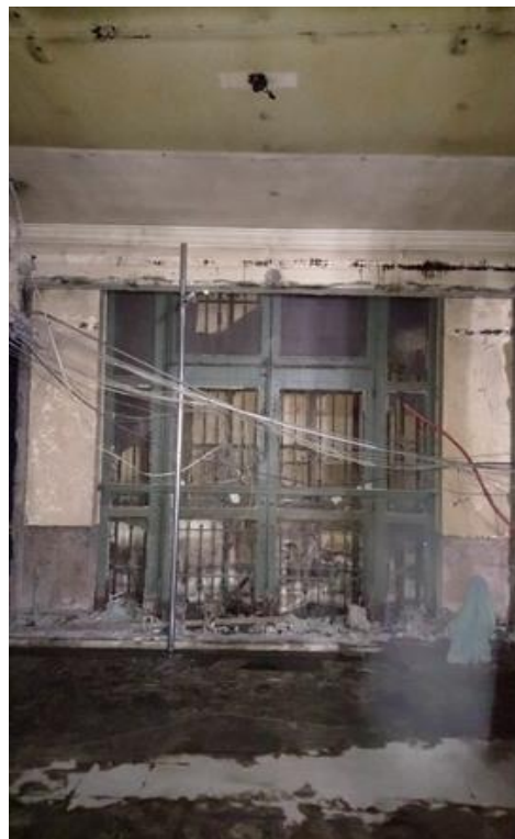
Revealed along Calle Juan Luna are the original entrance doorways to the banking hall. These are provided with hard wood frames and jambs supporting grilles and glazing. Opening inwards, these doors were sealed off when the mezzanine floor was added. Left: Door along Grid C-D. Bottom: Door along Grid D-E
