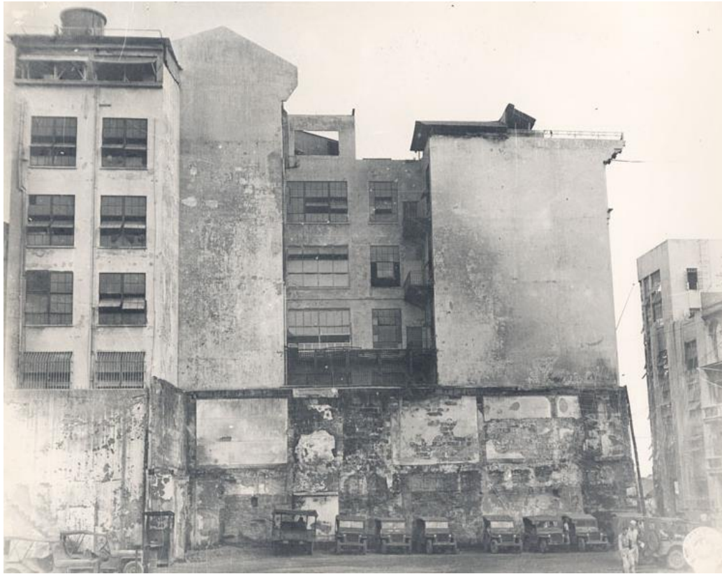
Post Liberation 1945 side picture of China Banking Corporation Building. Shows burn marks on retaining wall.
