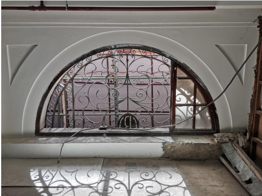
The lunette grillwork along Calle Juan Luna are protected by operable wooden and glass panels. The wooden frame along Grid D-E needs to be restored.
