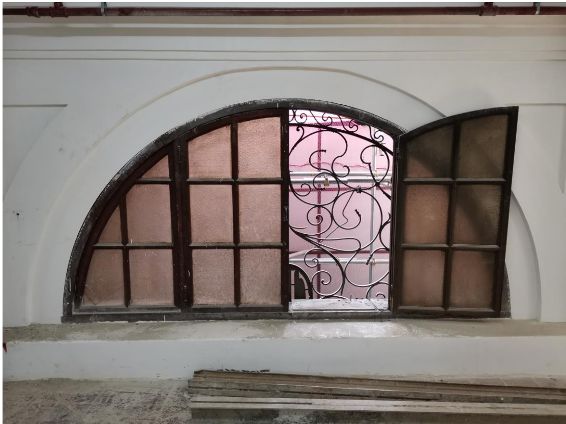
Lunette along Grid C-D still with its original glass framed panels.
