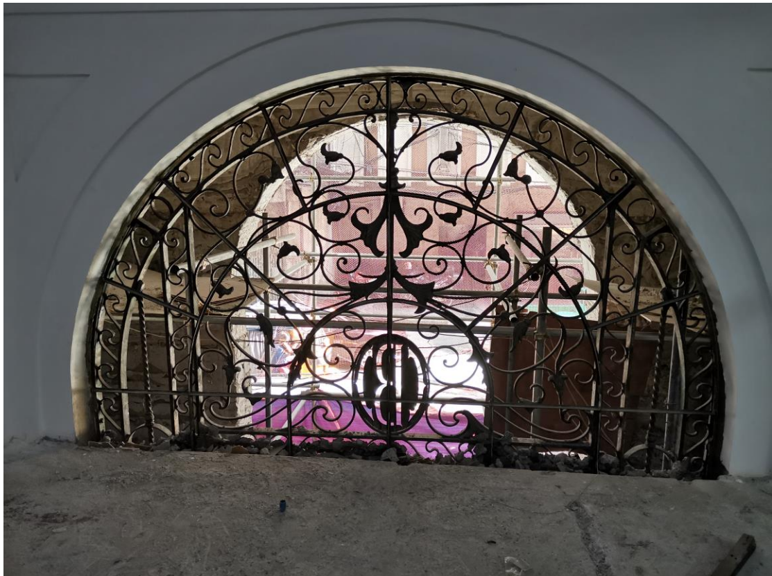
Grill work on the lunette along Grid 5-6 of Calle Dasmariñas. The Banks initials are emblazoned in the central escutcheon surrounded by curlicues, rosettes, scrolls and other romanticized grills.
