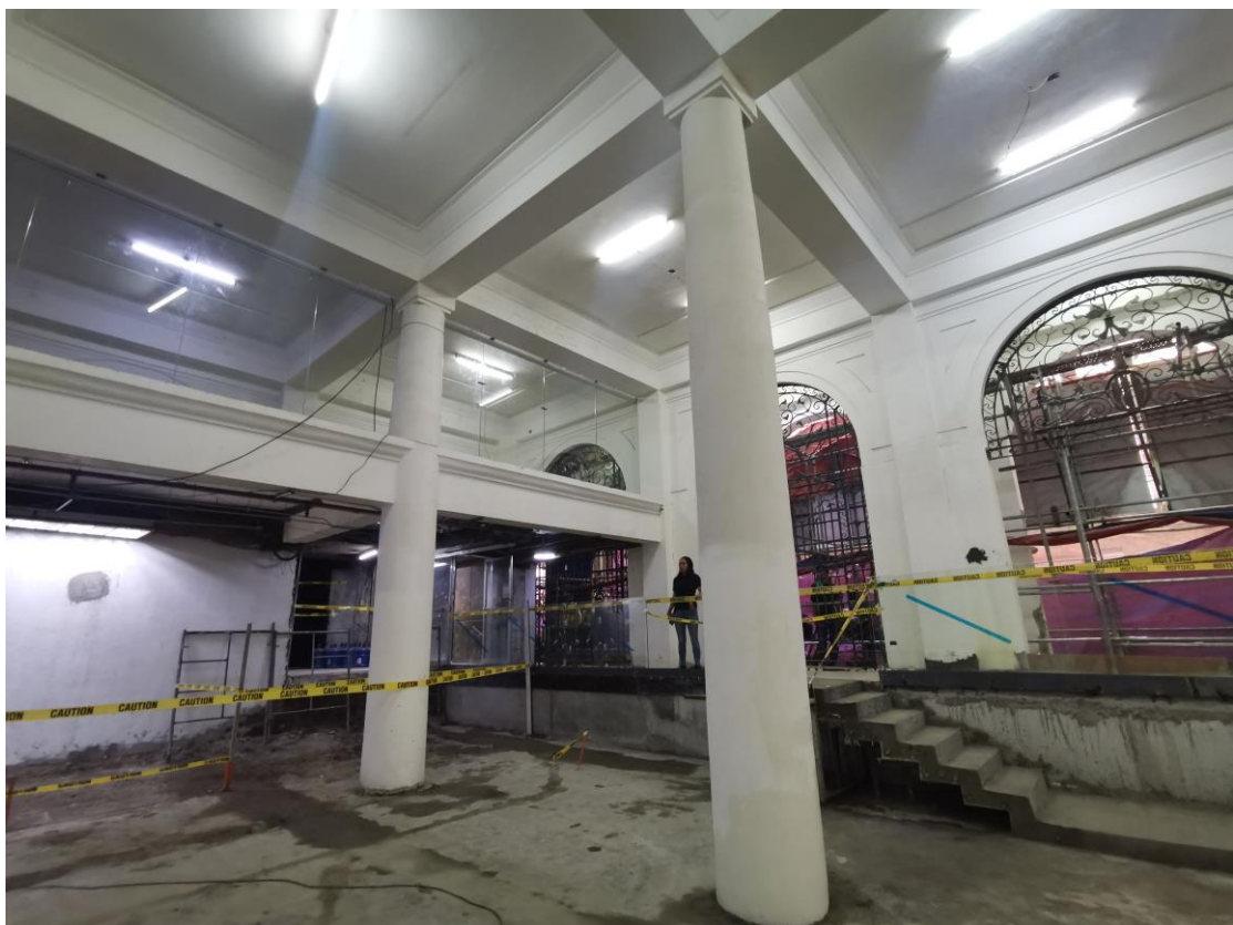
The elevated pathway links the banking hall with the elevator lobby to the left.
