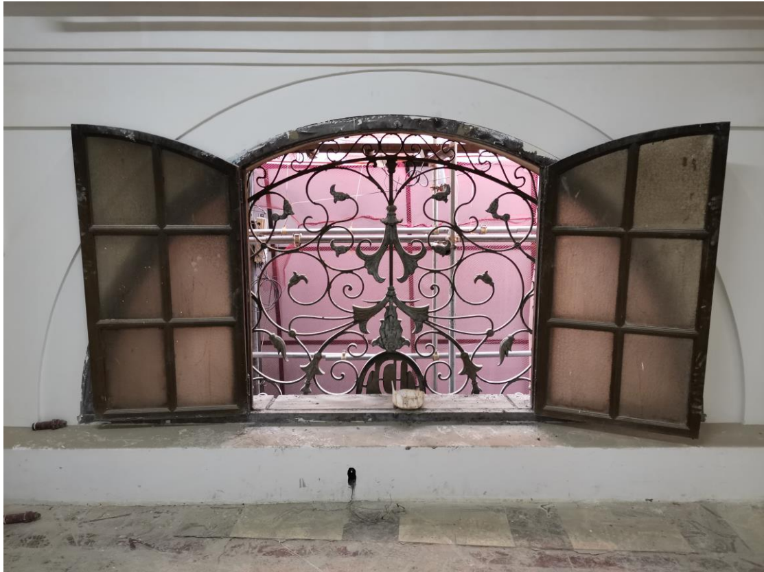
Lunette along Grid B-C with intact operable wooden windows.
