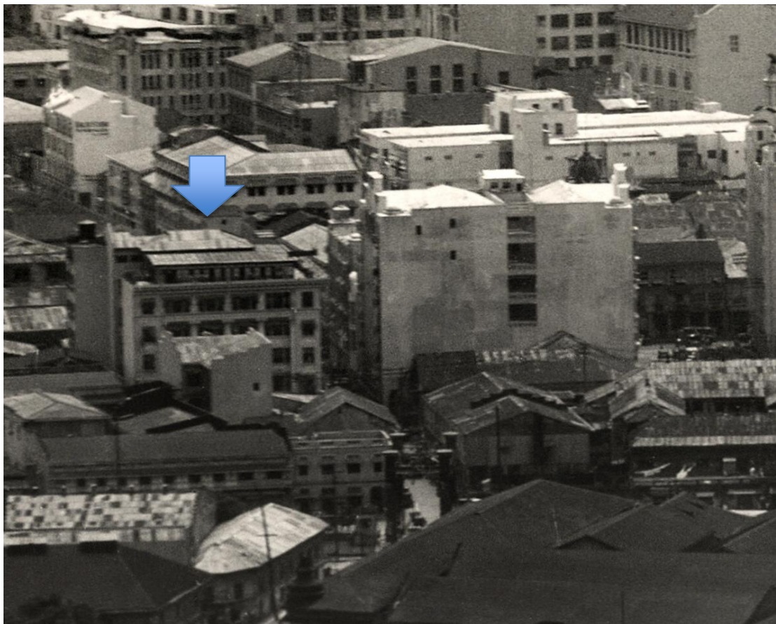
China Banking Corporation in August 1932. Aerial Photographs from the War Department US Army Air Forces, US National Archives. Picture shows 6 th floor pavilion with window and door placements. Visible as well is the 6 th floor hipped roof with lateral aprons.
