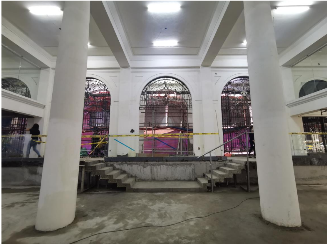
The new entrance to the restored banking hall along Calle Dasmariñas. An elevated platform connecting the new entrance to the previous provides a seamless link between one and the other. Sadly, with the decision to provide a new access the inevitable compromise had to be undertaken regarding the lower portion of the grill work, which was entombed with the additional platform.
