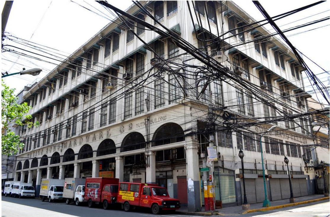
Yutivo & Sons Hardware Company building today. Like China Banking Corporation, the architectural language used in its façade is similar to those seen in the latter. Stately arches line the buildings arcade supporting above it grooved pilasters instead of rounded columns. But like the latter, the building also follows a tri-partite classic formula of base, shaft and capital, with the capital of this building being a simplified bracketed cornice.
