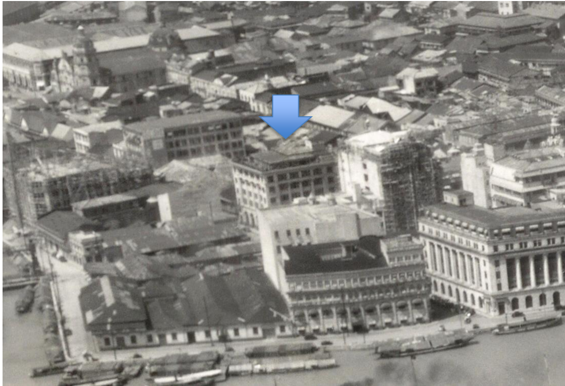
Aerial Photograph of 1935 showing CBC building at center with Berenguer-de los Reyes building (situated in front) still under construction.
