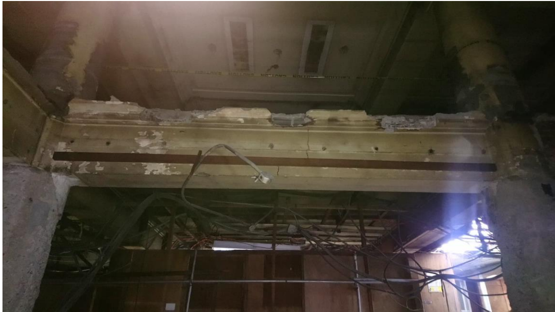
Damaged Cavetto mold seen on the mezzanine floor.
