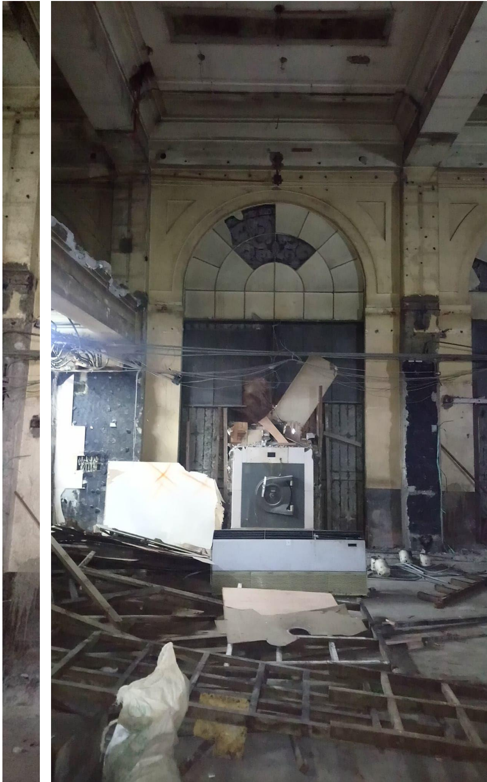
The third opening along Calle Dasmariñas with parts of the glazing gone. Showing the extent of cement filling on the grillwork. Also showing is the wooden jambs supporting the panels.
