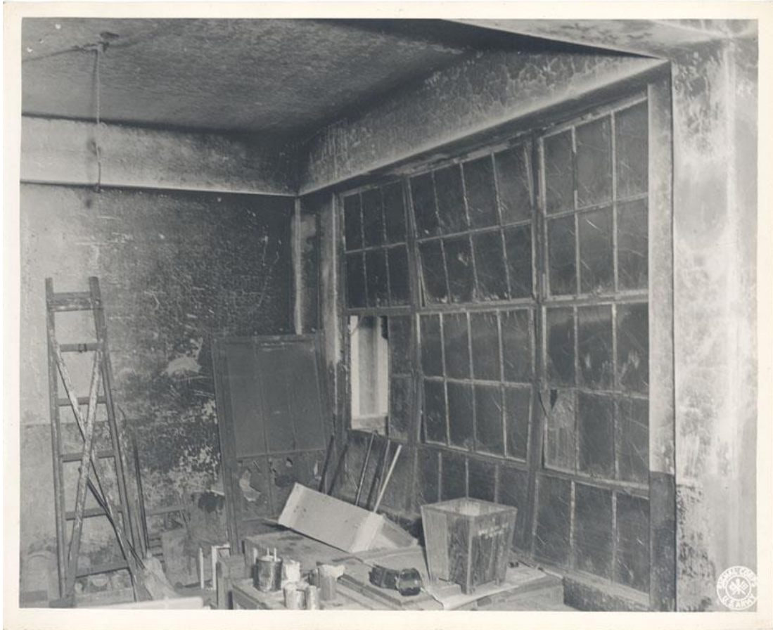
Left: Unidentified war damaged room inside the building. From the annals of China Banking Corporation: "The havoc and destruction caused by the battle for the liberation of Manila during the early parts of 1945 did not spare the bank. Extensive damage was caused to its building. Equipment and valuable records were destroyed. Its losses were so staggering that one despaired to think of it ever being rehabilitated."
