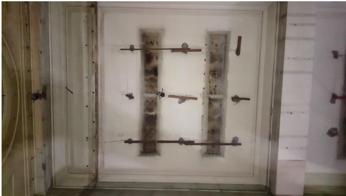
Each ceiling bay is lined with Cavetto molding except for the peripheral bays which has a further "C" shaped panel along the periphery.
