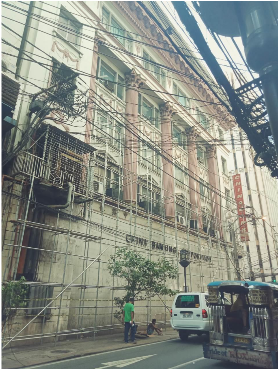
Scaffolding work being prepared at the start of the renovation work in July 2019. Marble tiles installed sometime in the 1970's hid the original arches. Cladding most likely was a result of the raising of the street level in Binondo area which increased in height by more than a meter in some areas.
