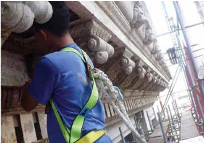
Worker meticulously cleaning, repairing, and restoring the building’s exterior moldings and ornaments.
