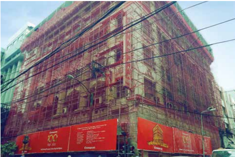
Steel scaffoldings surround the building for the painstaking work of restoring the ornate moldings, iron grills, and other exterior architectural details.
